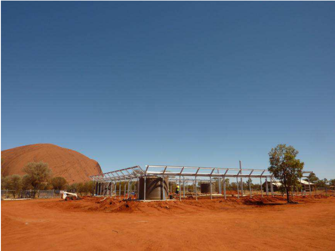
The Mutitjulu pool under construction
