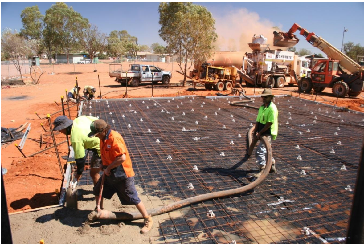
Contractors start pouring the concrete of the new Epenarra Church building
