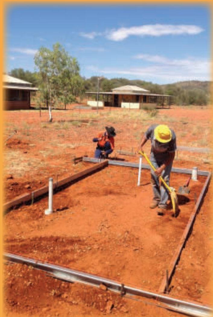
Building the new ablution block at Williams Well
