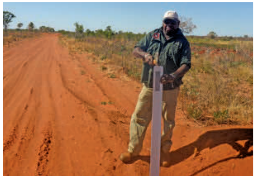
Jonathon Dixon installing a guide post.
