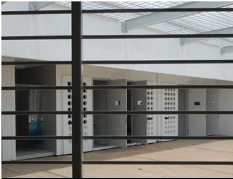
Cells inside the Don Dale Detention Centre, accused of "inhumane management". Photo ABC
