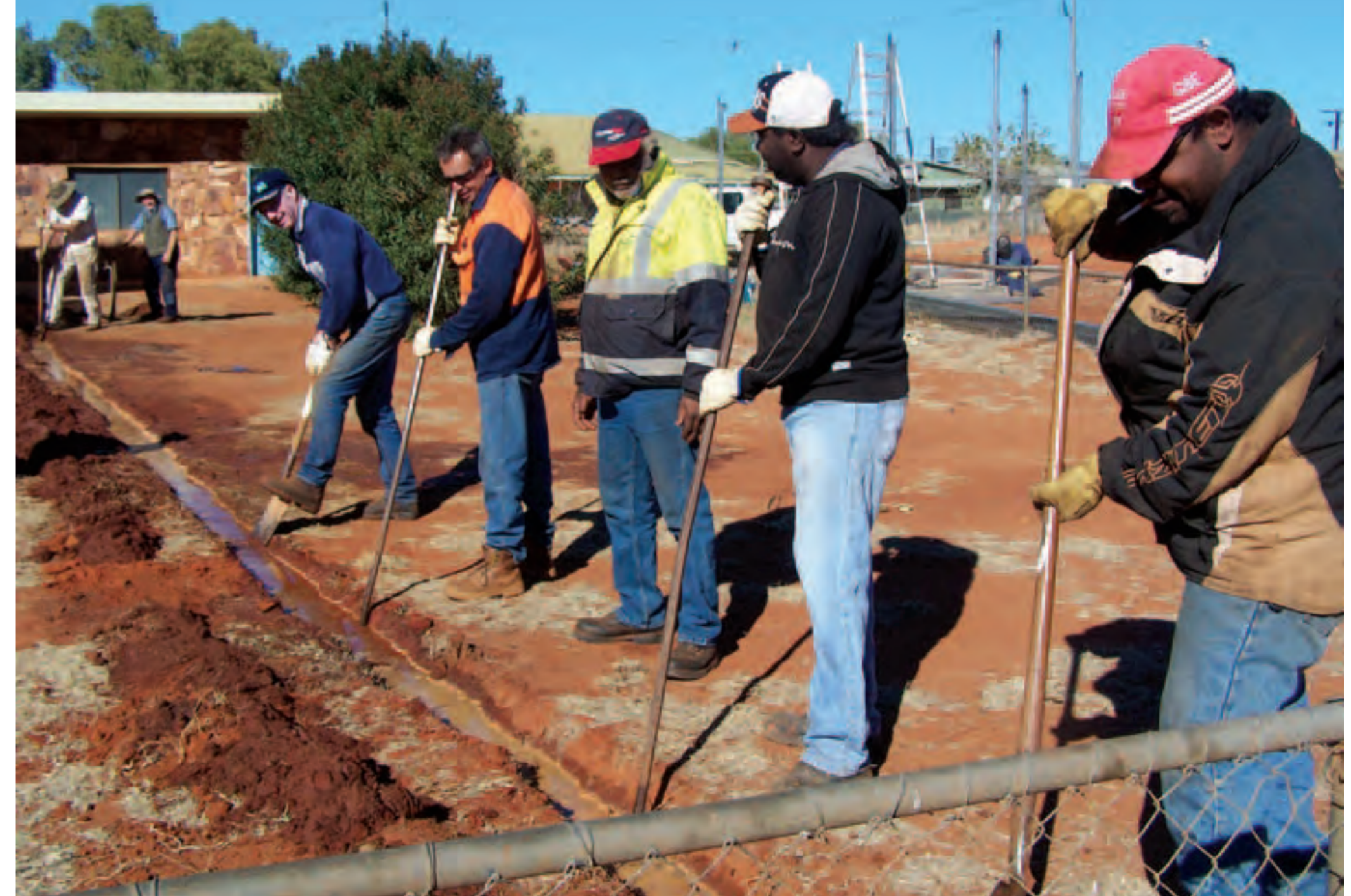
Installing water pipe at the Yuendumu Baptist church
