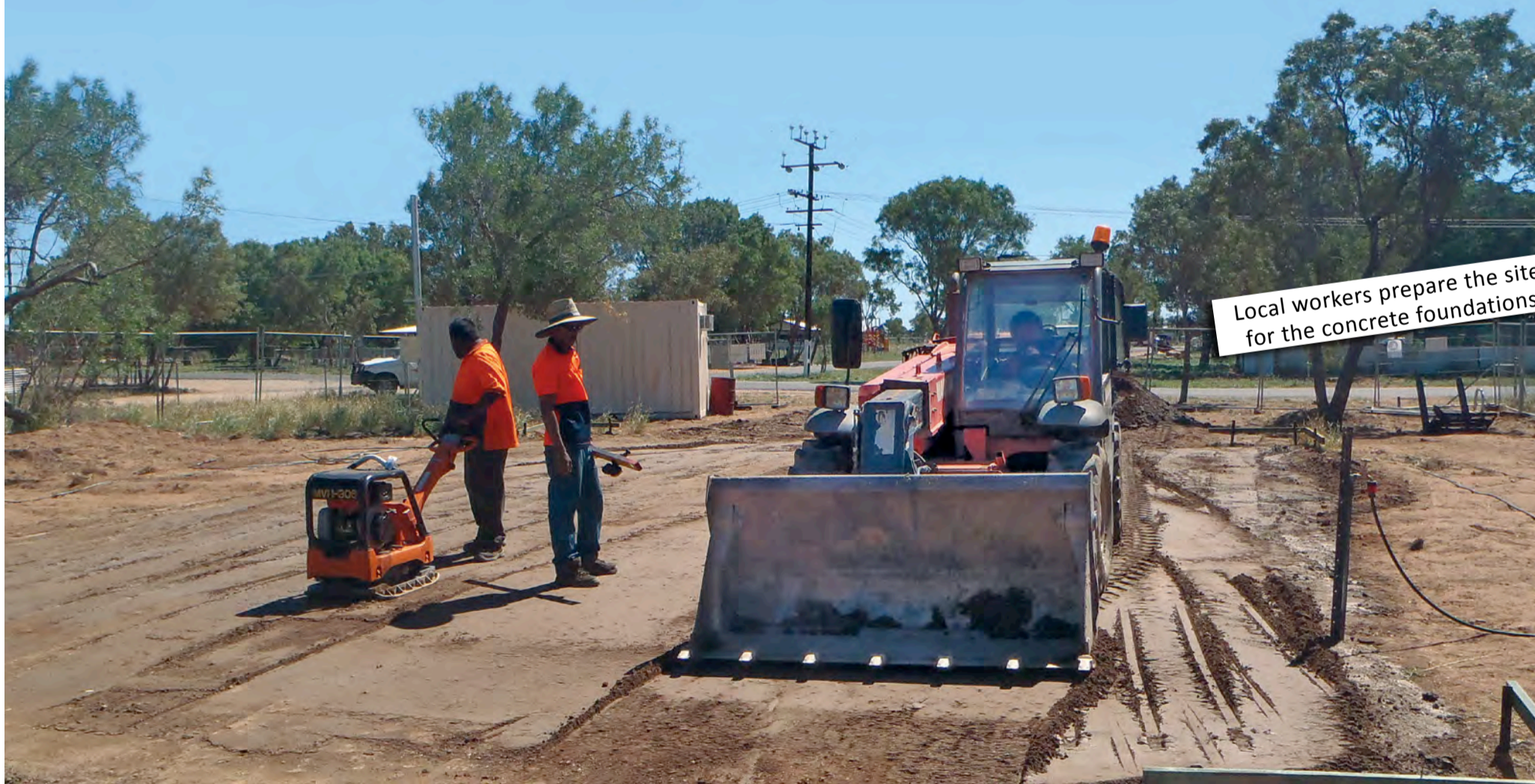
Anthony Petrick (left) compacts the site before the concrete can be poured. Peppi Drover (right) works on the church foundations.
