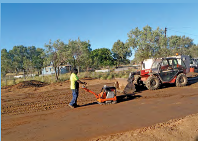
Anthony Petrick (left) compacts the site before the concrete can be poured. Peppi Drover (right) works on the church foundations.
